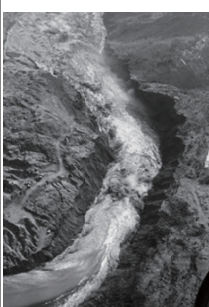
Breaching Tangjiashan landslide dam: Xu et al. (2009) Bull Eng Geol Environ 68:373–386
