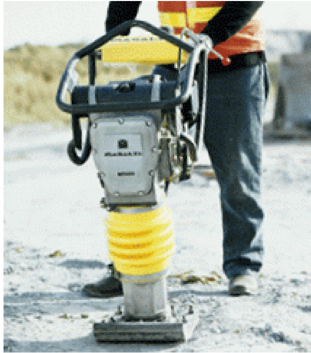
Fig. 1. Compaction of Soil with Vibratory Compactor
