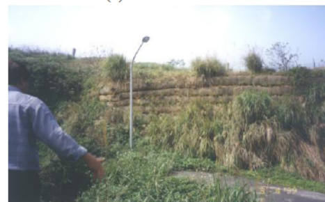
(b) Reinforced Retaining Wall at the Toe of Slope
