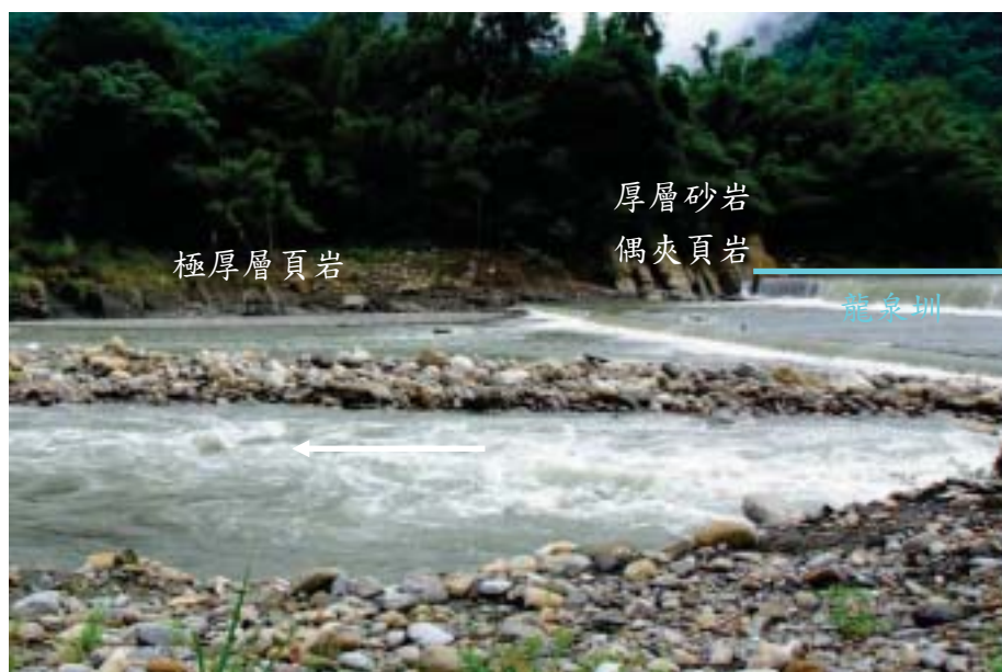
(b)堰體下方岩盤為厚層砂岩偶夾頁岩(232835, 2658010, N30E, 980806)
