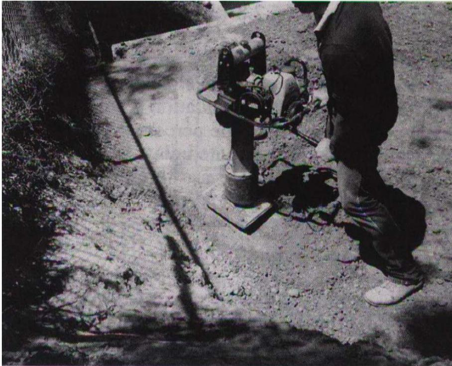
Fig. 1. Compaction of backfill using hand tamper (after Day, 1998)
