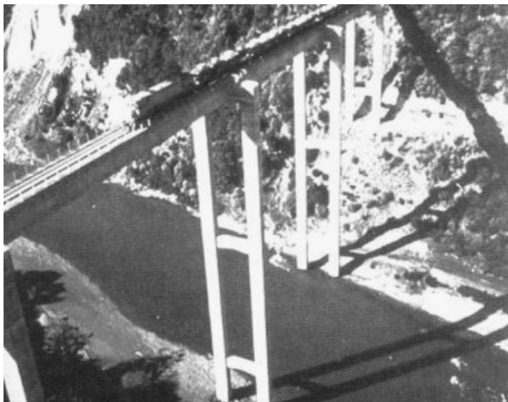
Figure 1. South Rangitikei Viaduct (New Zealand) [6].
