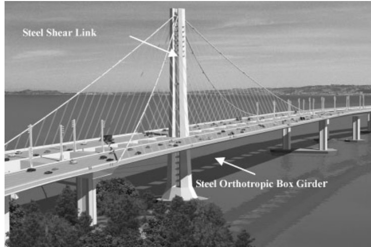
Figure 1. The new SFOBB East main span.
