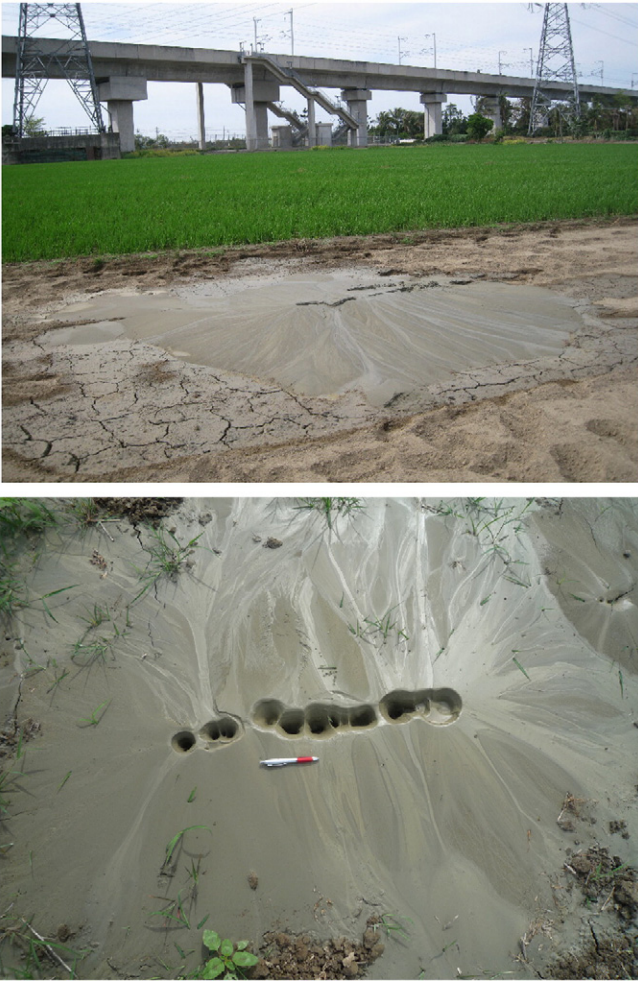
Fig. 2. Sand boils at Sinhua site (2010/03/05).
