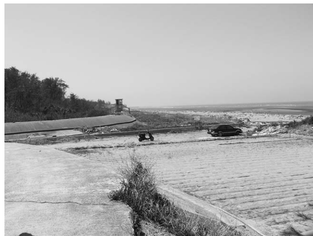
Figure 4. The beach and seawalls at Segment 20 of the Miaoli Coast.
