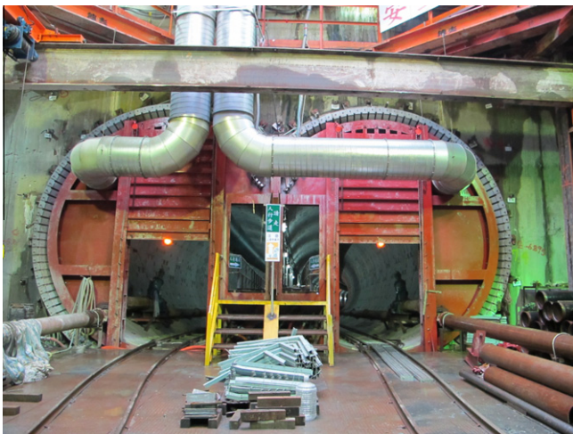
Fig. 8. South portal of DOT shield tunnel.
