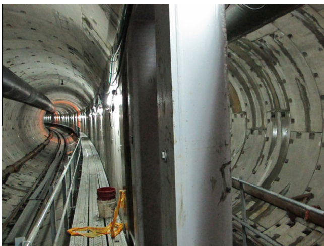
Fig. 9. DOT shield tunnels under construction.
