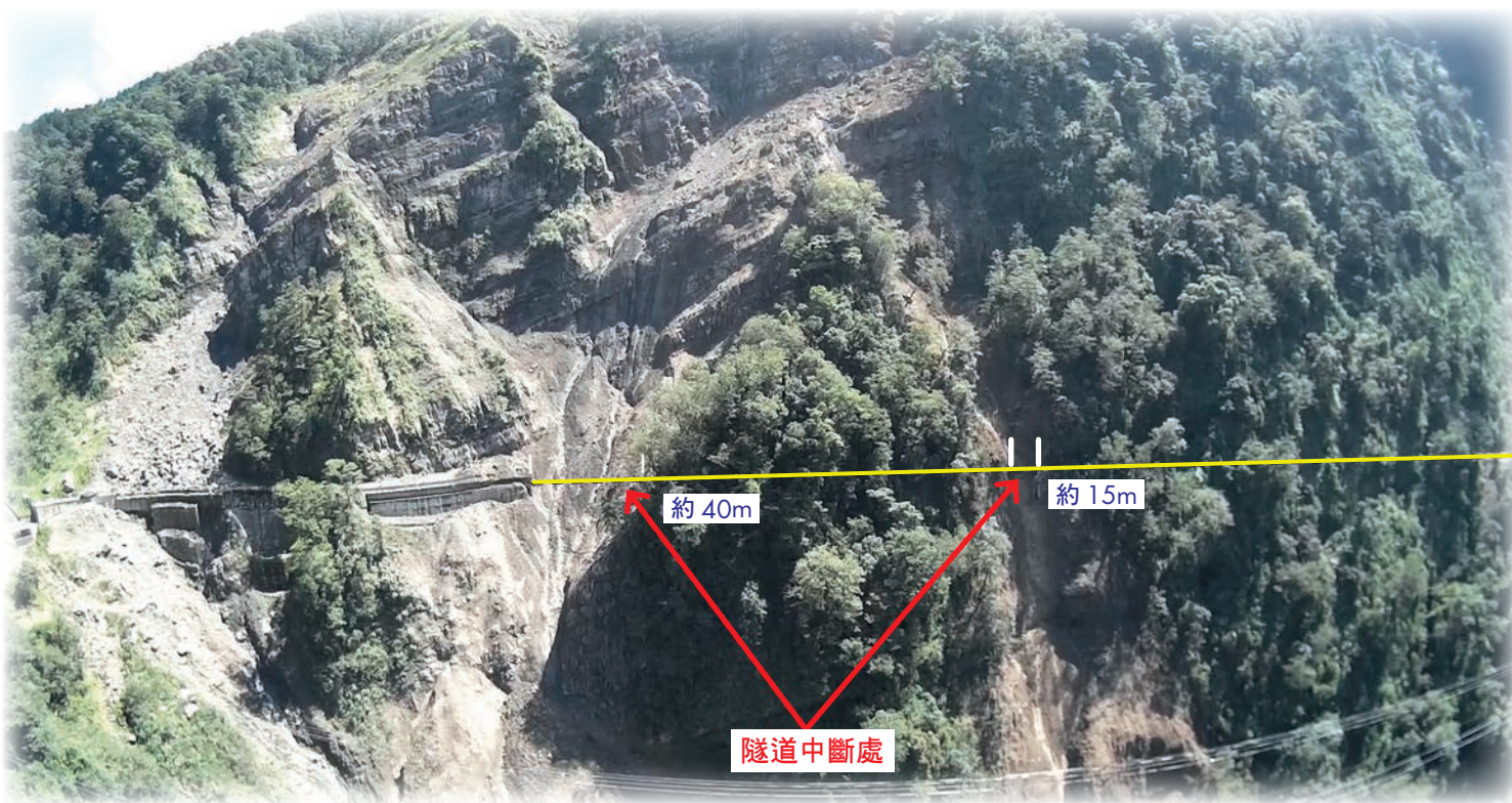
After Typhoon Dujuan struck, the tunnel was damaged by landslides and debris.
