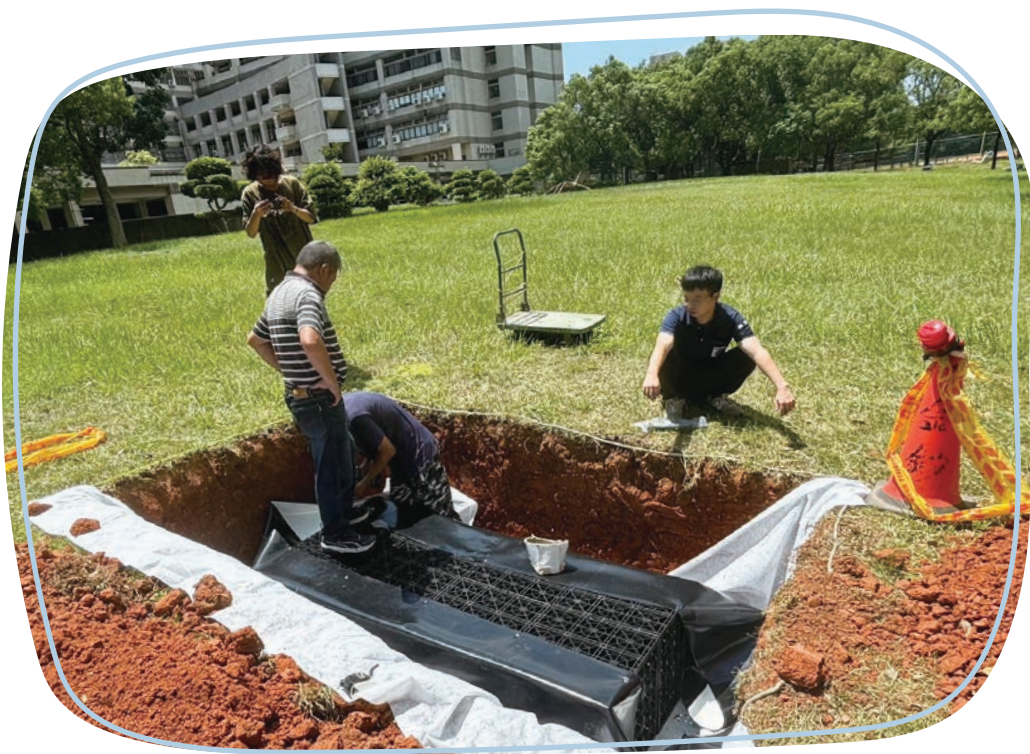
The black device shown in the photo is the water collection system, now installed beneath the lawn between Assembly Building 1 and Engineering Building 5 for testing.
