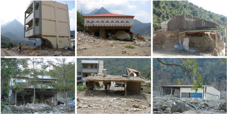
Fig. 3 Buildings damaged by debris flows during Typhoon Morakot 2009
