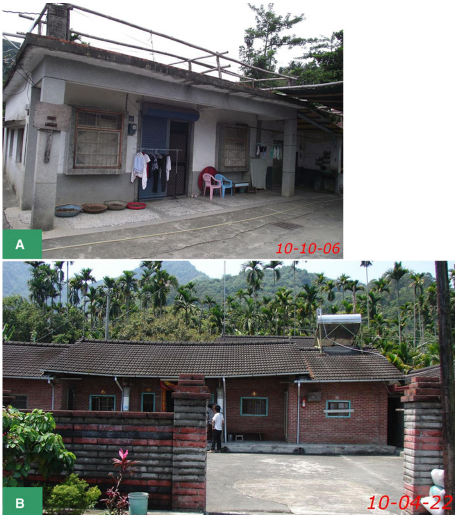
Fig. 7 Types of buildings: a reinforced brick: brick walls with RC column, beam and slab b brick: brick walls
