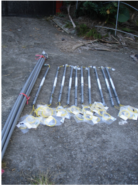
Fig. 9. PVC pipes and those with FBG piezometers enclosed.
