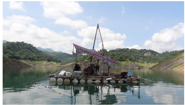
Fig. 7 The barge mount drill rig
