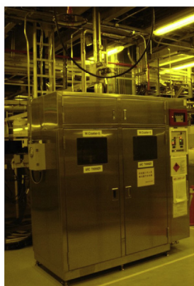
(a) Setting in the sub-Fab chemical storage cabinet (clean booth), chemicals were delivered to the clean room by the pump power of lithography process machine
