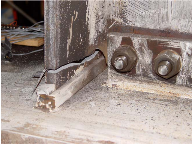
Fig. 14. Fracture of beam top flange of unreinforced specimen BUN.
