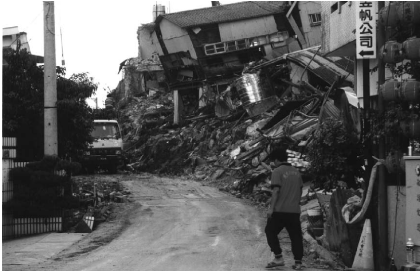
Fig. 7. Buildings damaged by the main rupture near the Chung-Cheng Park (1).
