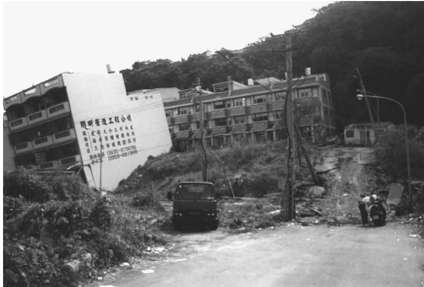
Fig. 3. Main fault near Park No. 1 Bridge. At ruptures along foot of the hill and appears to be a thrust with a slight left-lateral component. The vertical uplift is 4–5 m and the apparent horizontal separation is 7 m.
