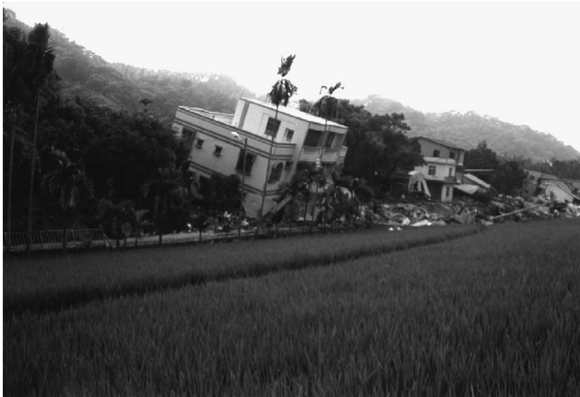
Fig. 8. The buildings damaged by the main rupture near the Chung-Cheng Park (2). The main rupture extends along foot of the hill.
