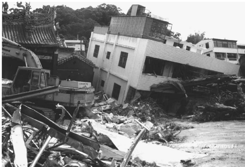
Fig. 10. Buildings damaged by the main rupture near the Chung-Cheng Park (4).
