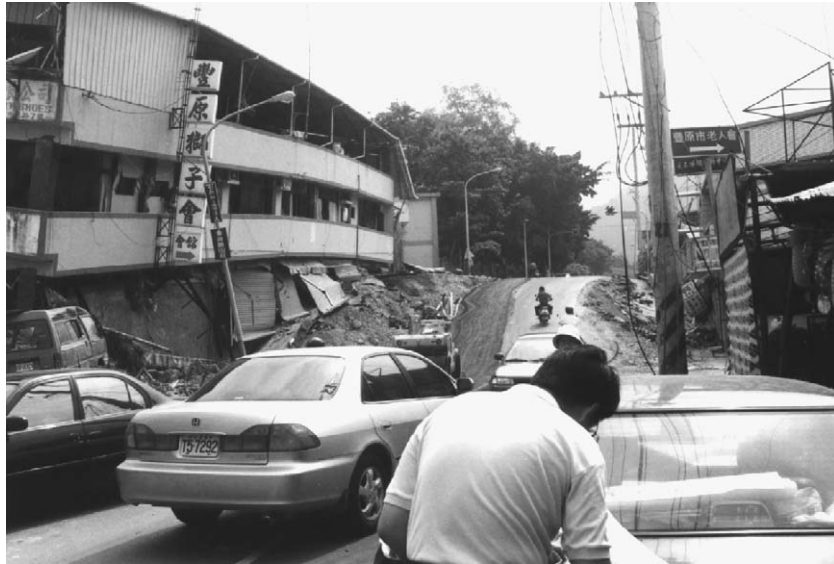
Fig. 9. Buildings damaged by the main rupture near the Chung-Cheng Park (3).
