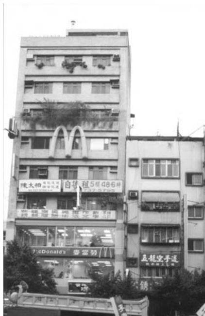
Fig. 1 Buildings without proper separation distance (Keelung Road, Taipei)
