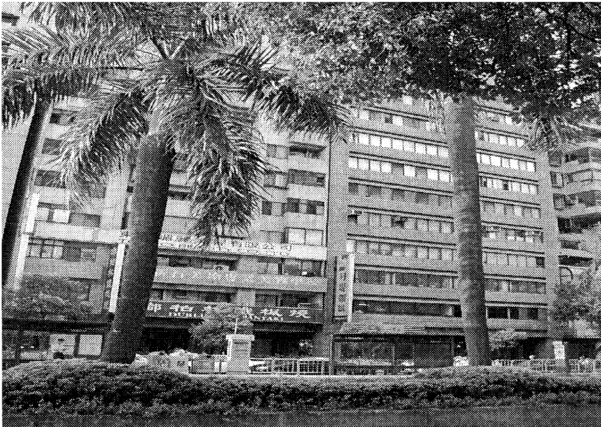
Fig. 4. Typical street buildings at site A.
