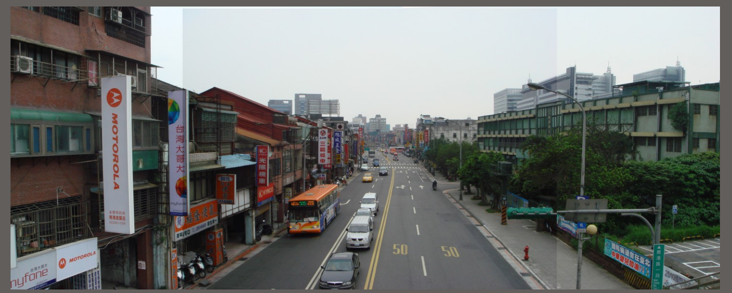
Western View of Site
