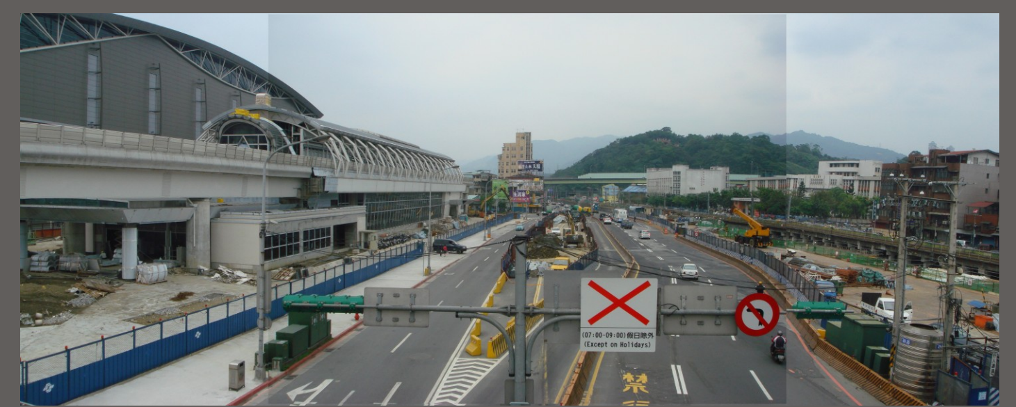
Eastern View of Site
