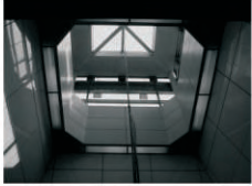
ORIGINAL SKYLIGHT WELL INTERIOR
