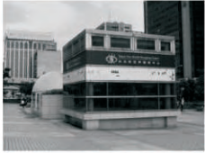
ORIGINAL SKYLIGHT WELL EXTERIOR
