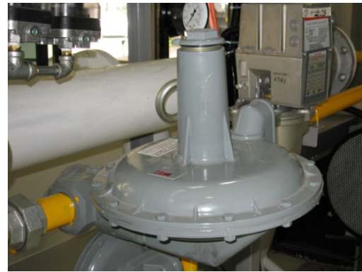
(b) Pressure regulating valve
