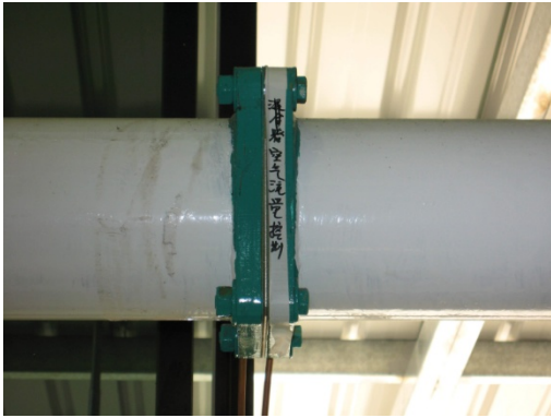
(a) Orifice plate
