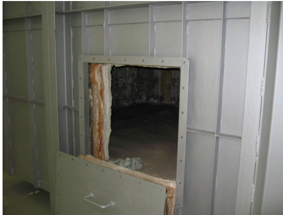
(c) Manhole cover
