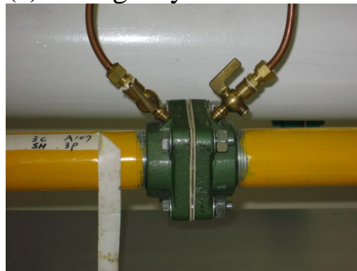
(c) Orifice plate
