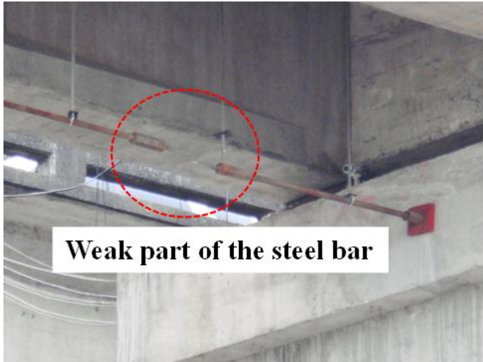
Figure 6.13 Weak part of the steel bar
