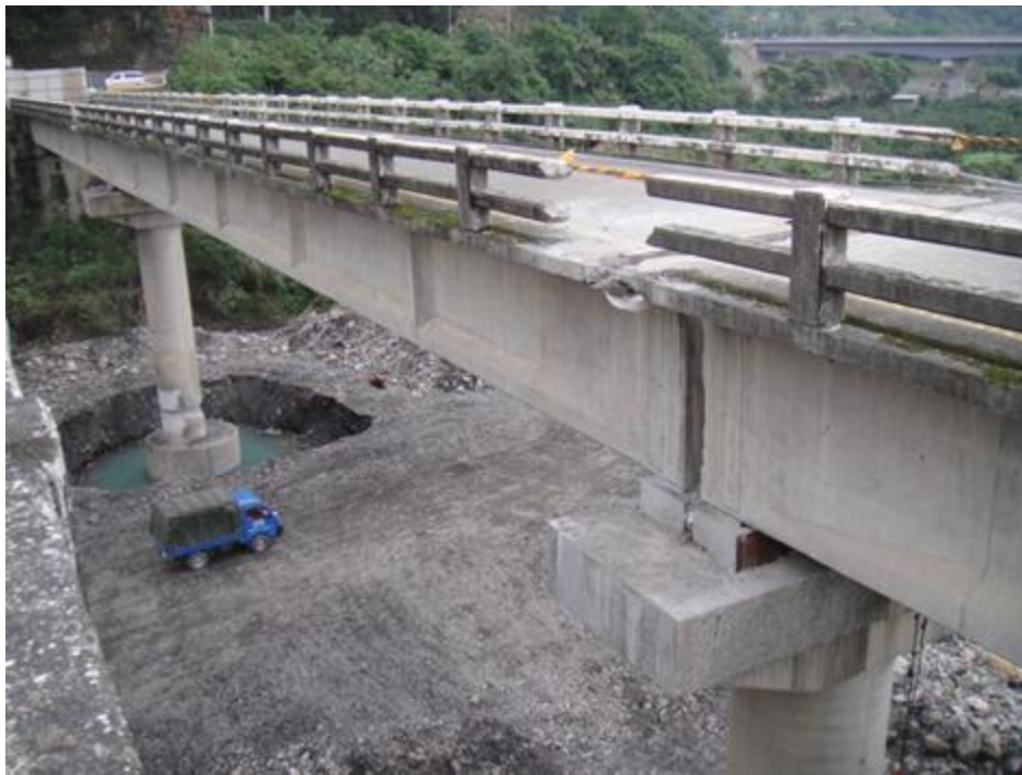
Figure 6.12 Photo of Nioudou Bridge
