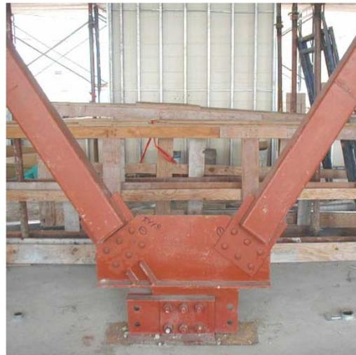
Friction damper in chevron bracing (inverted)
