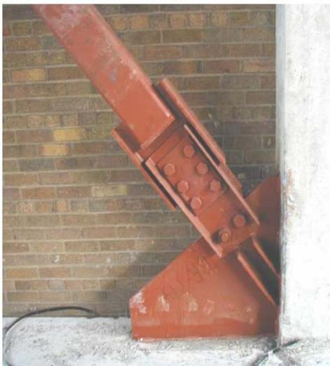
Friction damper in single diagonal bracing
