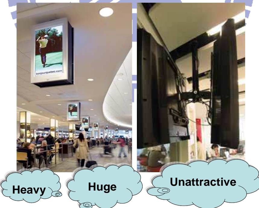
Fig. 7-8 Ineffective applications of two conventional sets of single-sided LCDs installed back-to-back.
