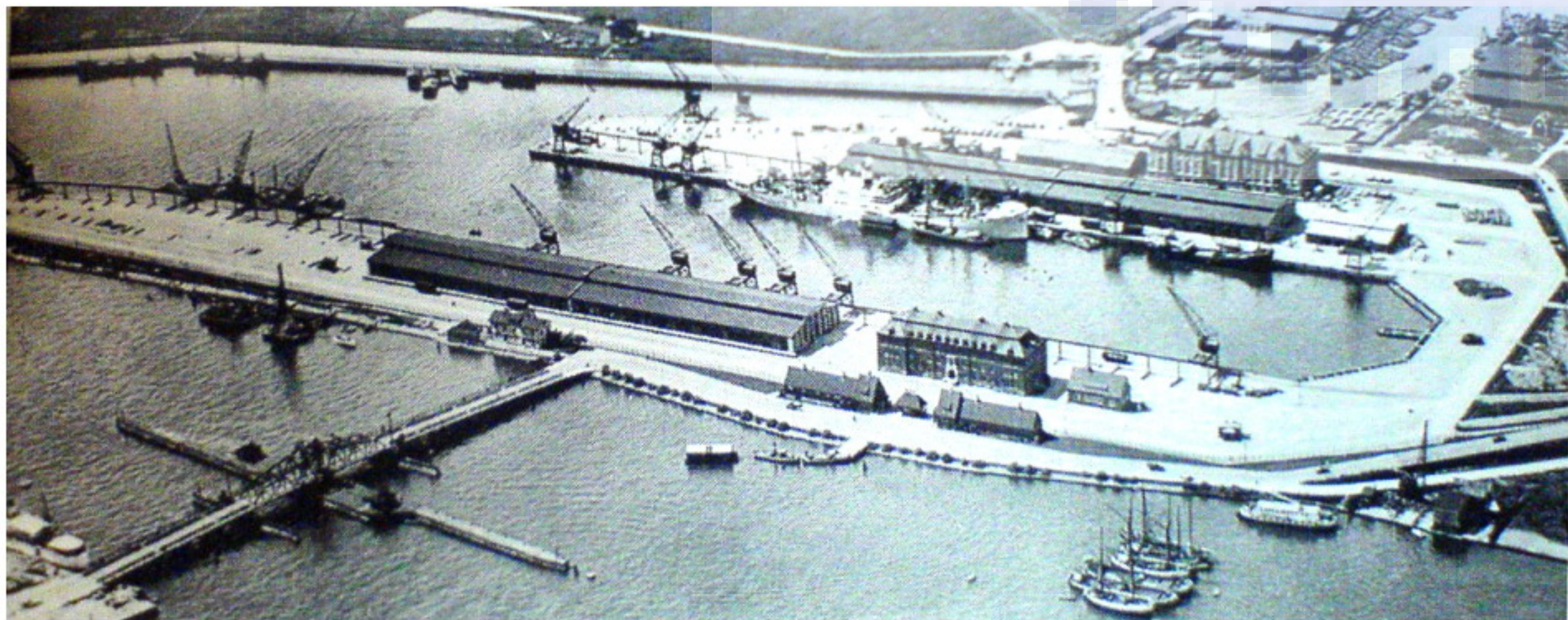
Frihamnen in the 1930s. In the foreground the old bridge (Hisingsbron) over Göta Älv.
