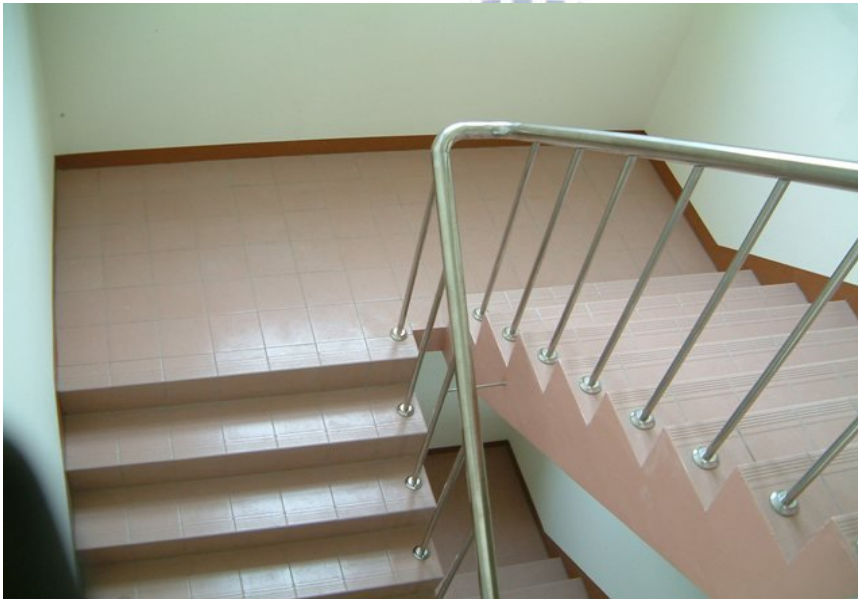
Figure.7 Stair Well of the Building
