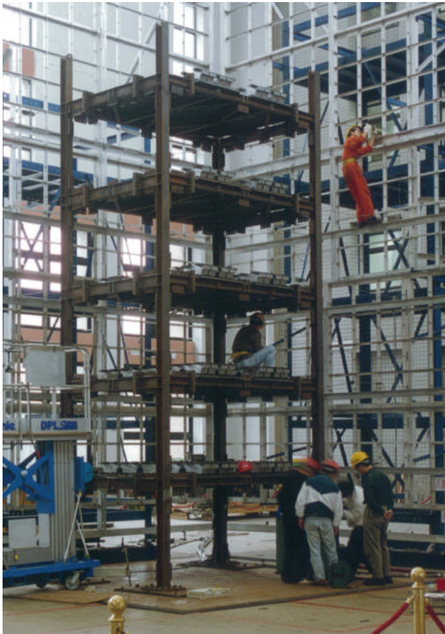
Figure 4.5 A photo of the five-story steel frame in NCREE
