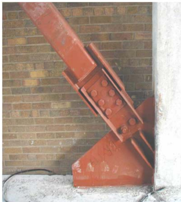
Friction damper in single diagonal bracing
