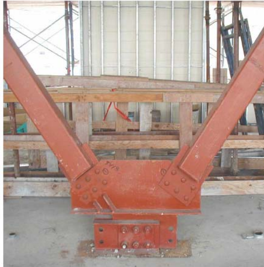
Friction damper in chevron bracing (inverted)
