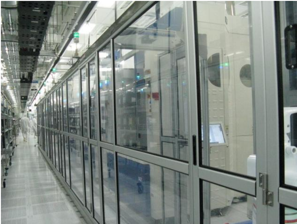
Figure 3.1: Class-100 Clean Room.
