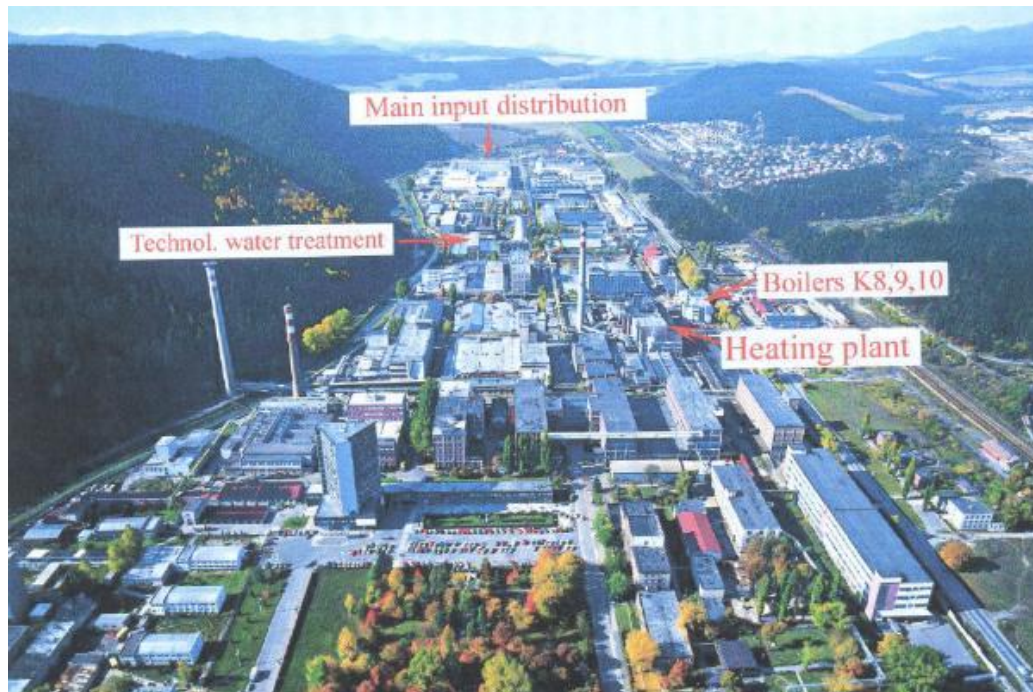
Figure 5.3: Technological Centers of Chemosvit Energochem a.s.
