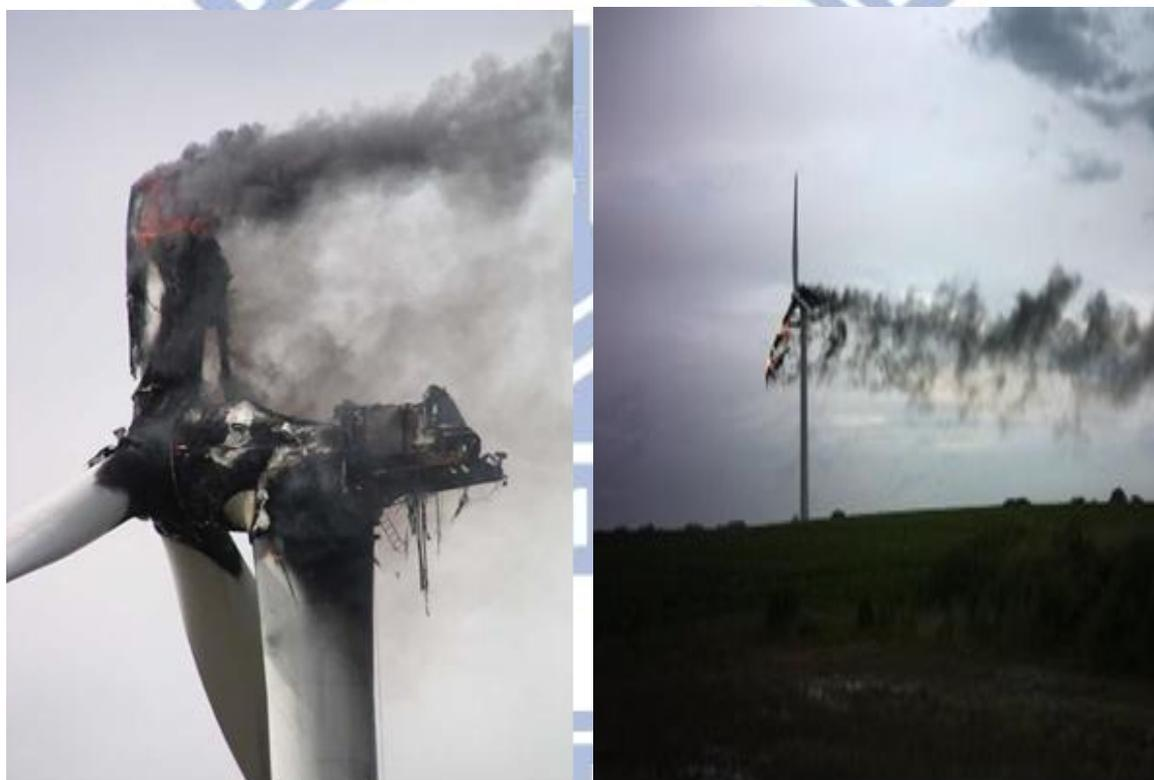
圖 5 Fire after lightning struck a 2 MW wind turbine in 2004 (Image source: HDI/Gerling)
