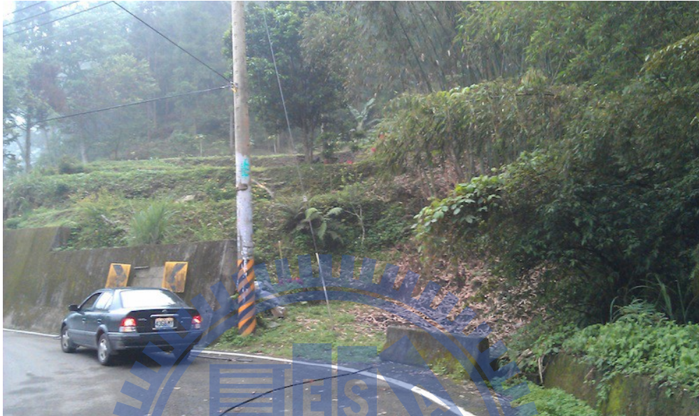
Illustration 19: The cement wall beside the green car and the power pole was designed to stop the flooding from the re-entrant.
