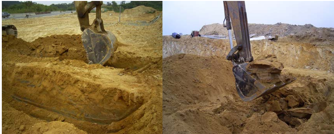
(a) 挖兩道深溝
