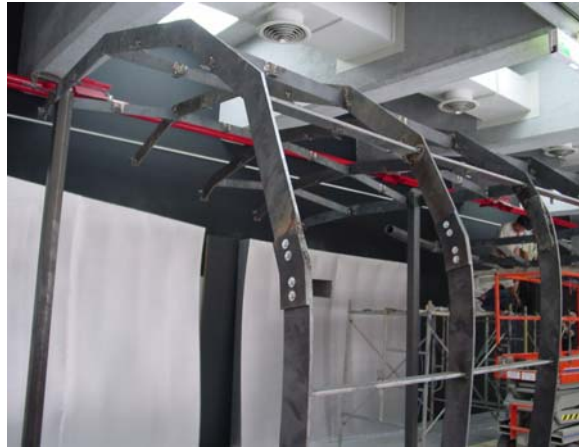
Figure 3.20 北美館數位展品可拆卸骨架
