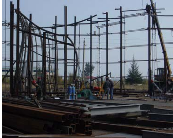
Figure 4.28 放樣現場尺寸核對預組裝尺寸
