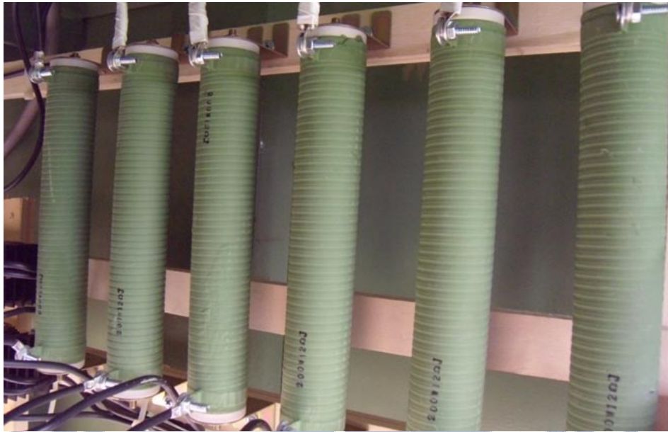
Fig. 4.11 Power type wire wound resistor
