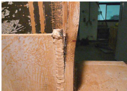
Figure 10. Specimen SP3 test observation (after second test).
