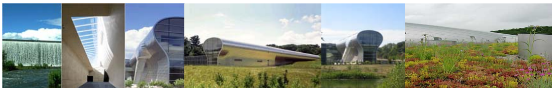
Figure 3-5. View of Whitney Water Purification Facilities and Park
