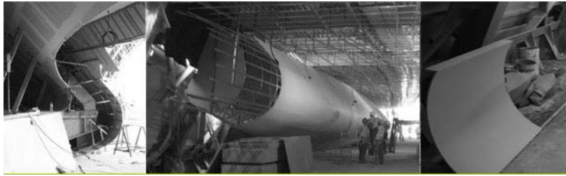
Figure 4-68. The Glass Fibre Reinforced Concrete (GRC)
