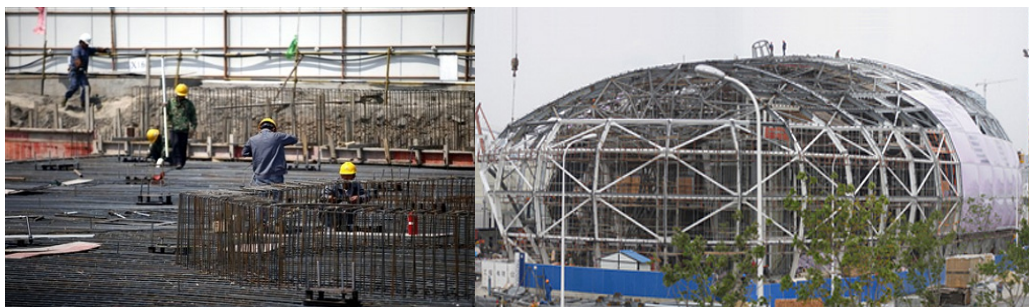
Figure 4-88. The Steel Frame Structure
