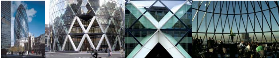
Figure 3-1. View of Swiss Re Headquarters
