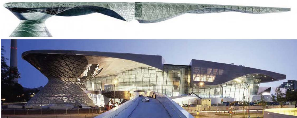
Figure 4-43. The Continuous, Overhanging, Tornado-like Roof
