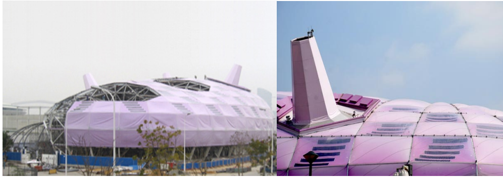
Figure 4-93. The ETFE Double-layer Pillow Membrane Envelope
