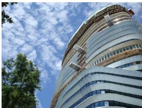
Figure 4-112. The Horizontal Fins around the Building are Installed after the Construction
