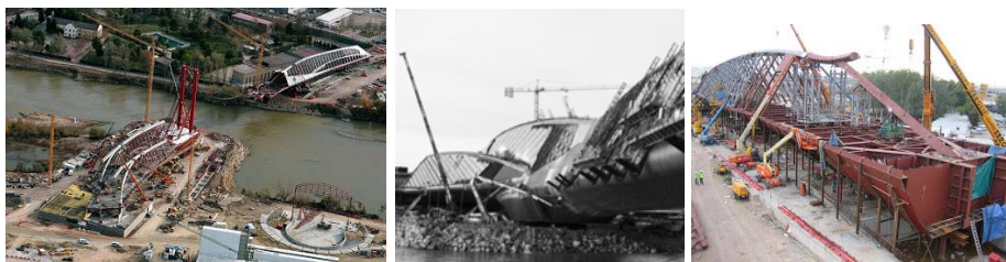
Figure 4-64. One of the Greatest Construction Challenges of the Entire Expo
