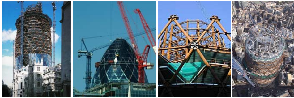
Figure 4-4. Swiss Re Headquarters under Construction
