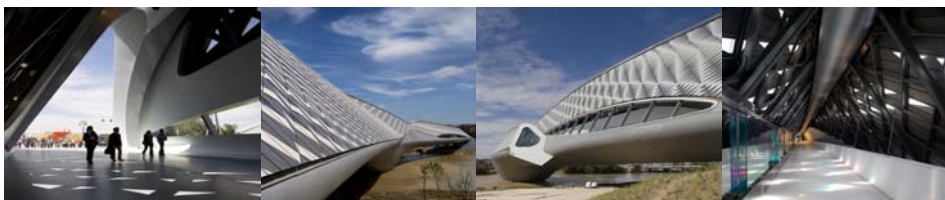
Figure 3-6. View of Zaragoza Bridge Pavilion
