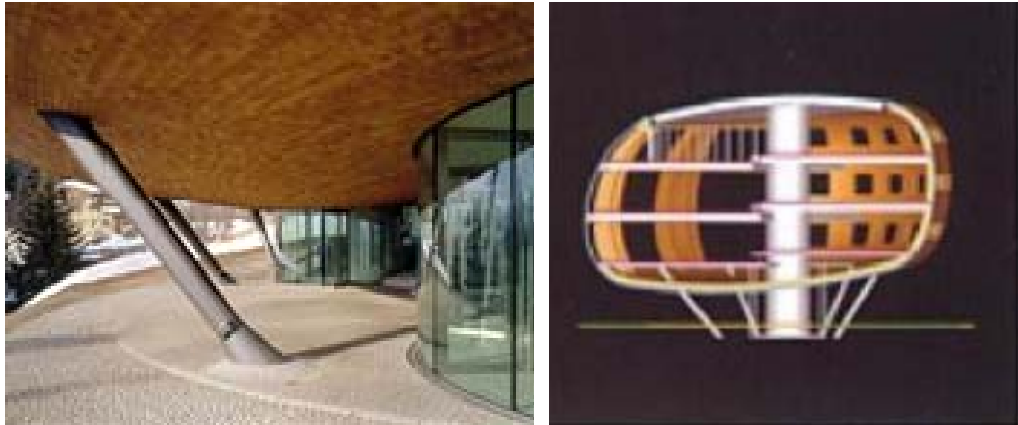
Figure 4-18. View of Steel Piloti
