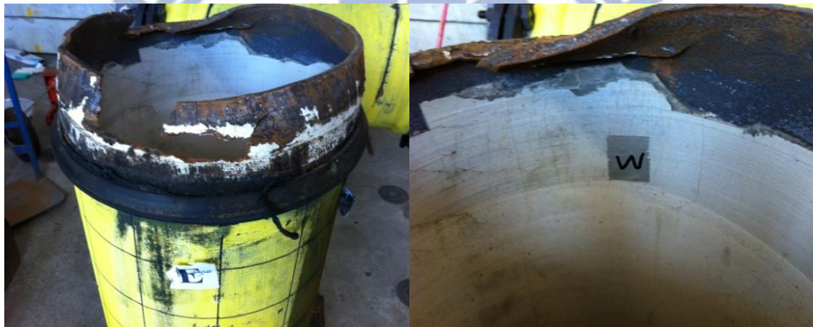
(a)承口端鑄鐵彎曲破壞
