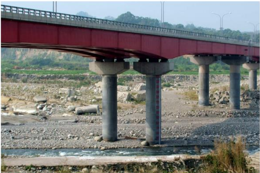
(b)水尺裝設情形(231607, 2689301, S45W, 980923)
