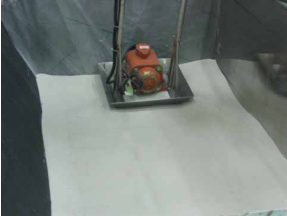
(a) Compaction of backfill by square compactor at H = 1.2 m
