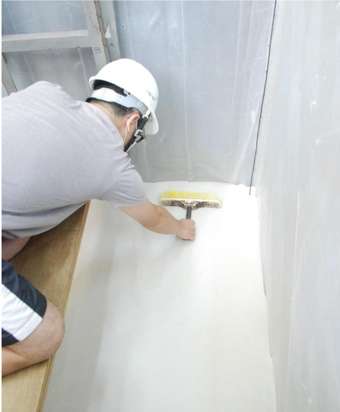
Fig. 5.6. Leveling of soil surface with a brush
