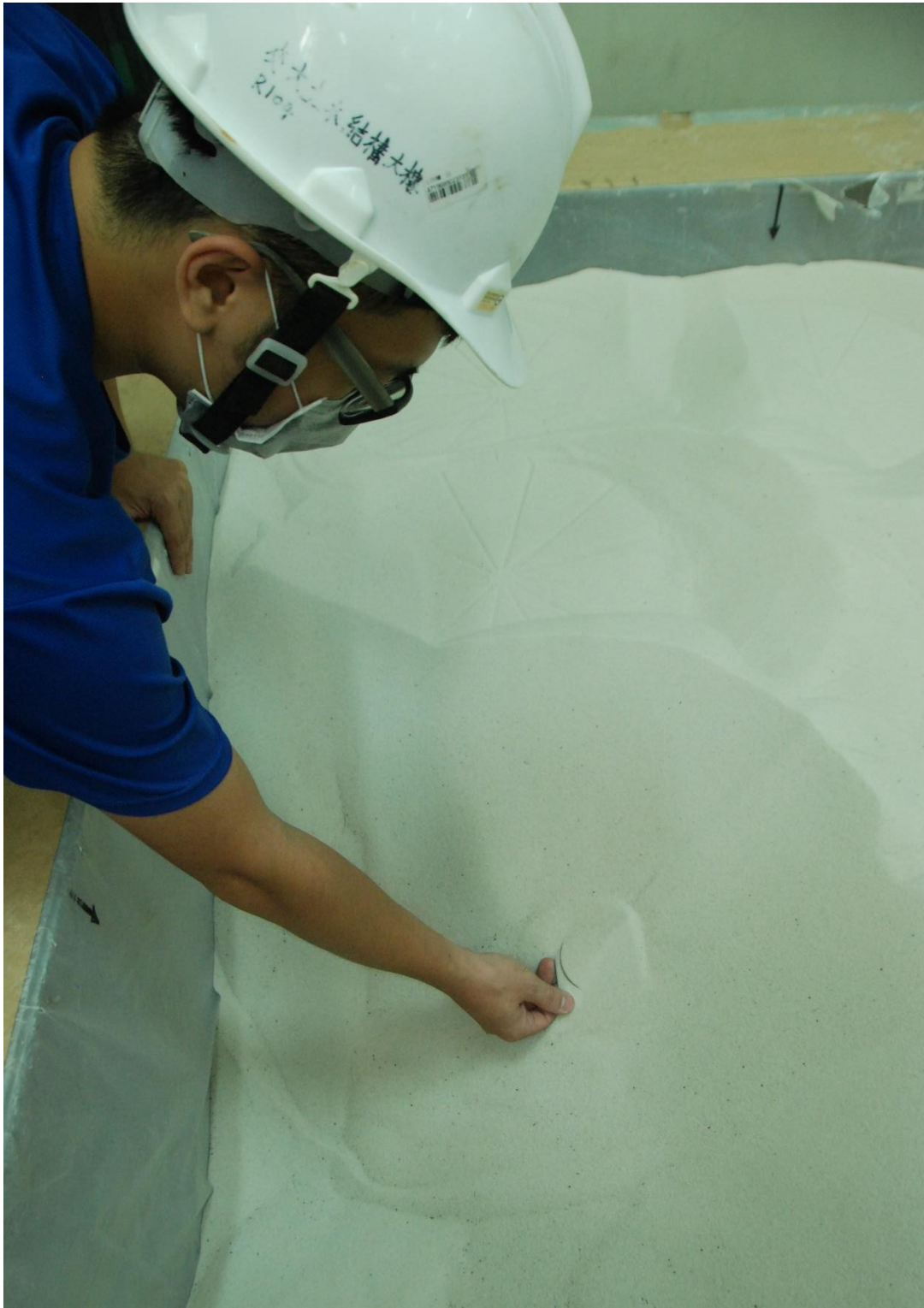
Fig. 5.19. Soil density cup dug out of compacted soil mass
