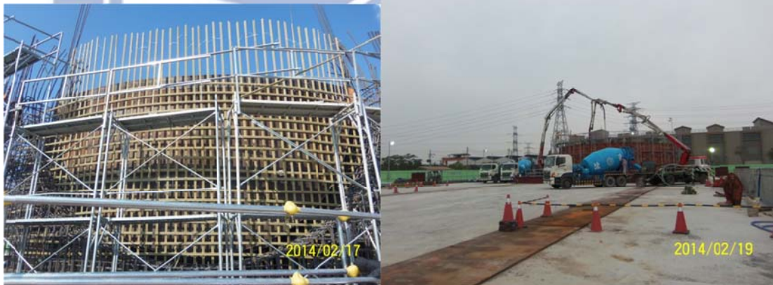
(a) 綁紮鋼筋
