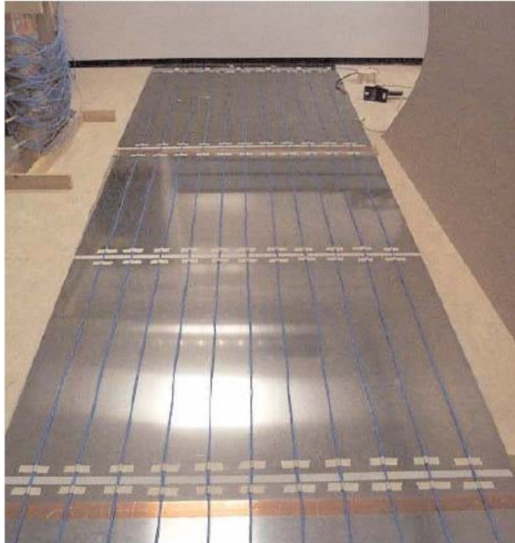
Fig. 2.3 Cable layout of unshielded twisted pair (UTP) [5, [6].
