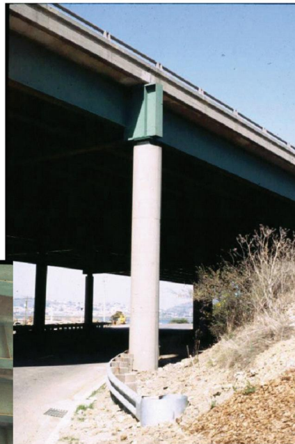
(b) Left: Replacement of existing steel bearing with lead-rubber isolator.
