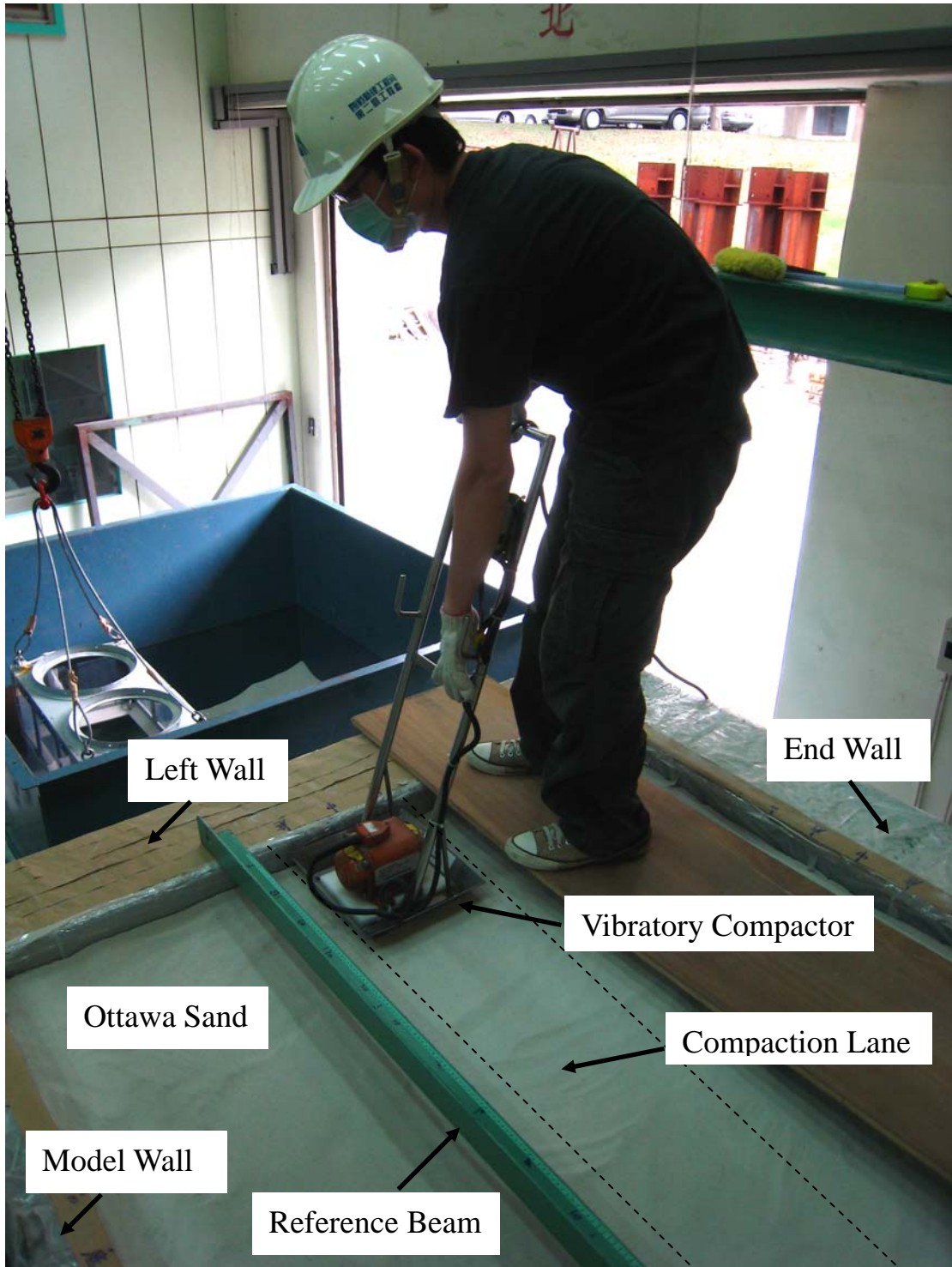
Fig. 6.2. Compaction on Surface of Backfill
