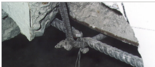
(c) 拉力筋斷裂
