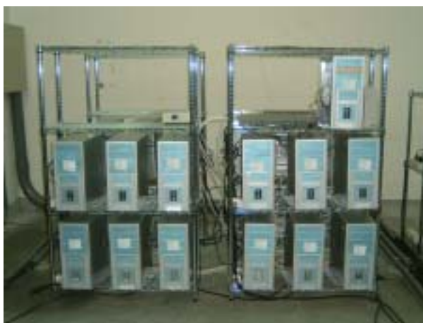
Fig. 2 23-node PC-Cluster system at MuST
